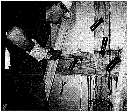
Figure 4.27: Vibration Through Access Holes
