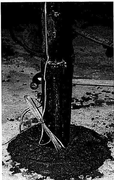
Figure 4.29: Installation of Shear Lug (Note Welded Joint)
