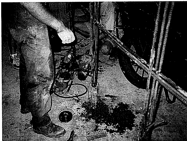
Figure 4.30: Vertical and Horizontal Strip Reinforcement Installed
