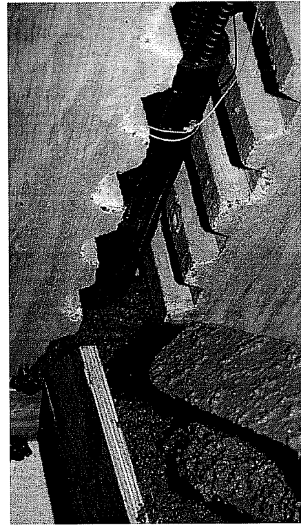
Figure 4.24: Grouting of Shear Lugs in Footing
